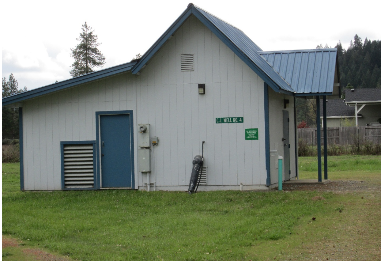
Figure 6.1.4-1 – Daisy Hill (Well No. 4) well house
