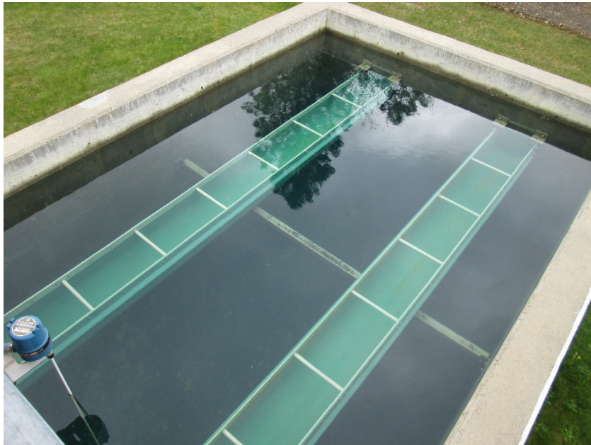
Figure 6.2.4-1 – One filter at the treatment plant.
