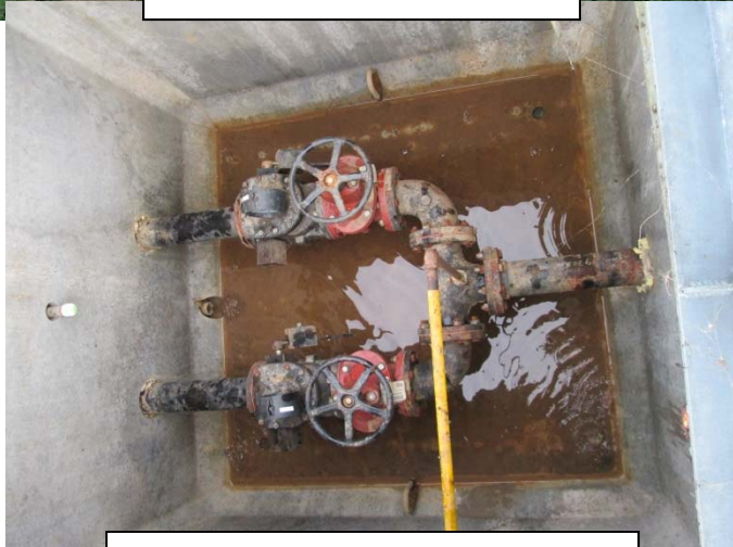
Figure 2.3.3c – Pomeroy View PS Forcemain Manifold
