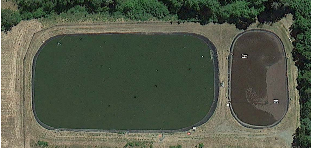
Figure 4.12.4a – Aerial Photo of Digester and Storage Lagoon
