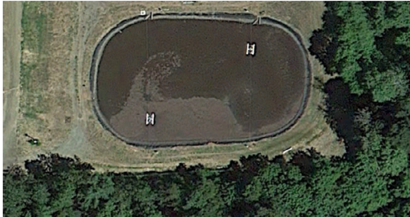
Figure 4.11.3a – Aerial Photo of Aerobic Digester
