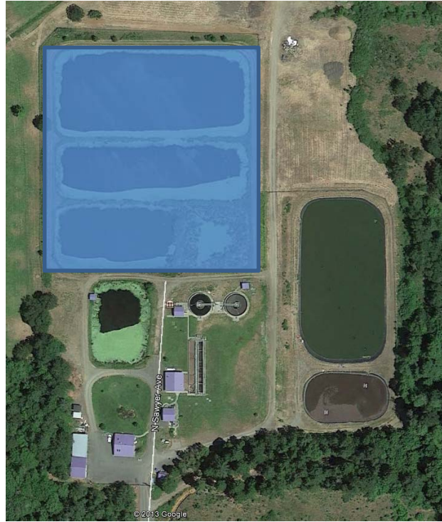
Figure 4.10.3b – Effluent Storage Basin
