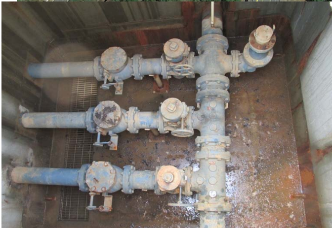
Figure 2.3.2c – North Loop PS Forcemain
