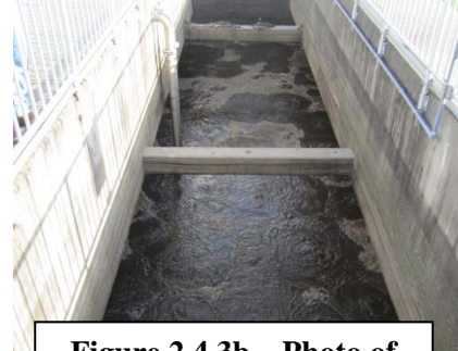
Figure 2.4.3b – Photo of East Aeration Chamber
