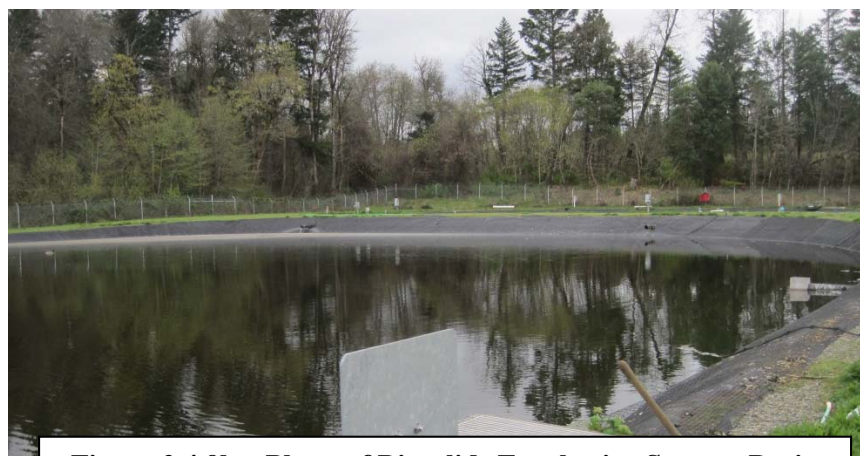
Figure 2.4.9b – Photo of Biosolids Facultative Storage Basin
