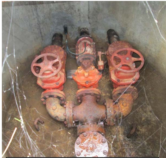
Figure 2.3.5c – Ranger Station PS Forcemain Manifold
