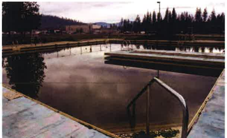
Looking South from the Cave Junction Pool
